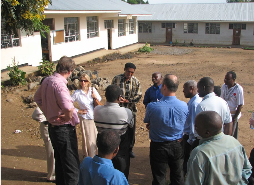
A new high school in Arusha, Tanzania. Notice the missing gutters; water flows away in the rainy season and then is lacking in the dry season. 2008
